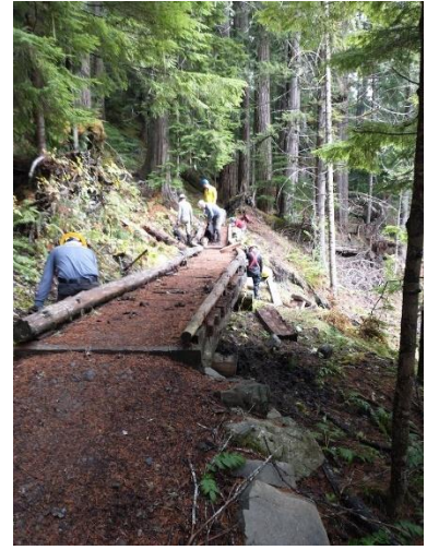
Shoveling in the muck; sawing old planks; clearing out the uphill ditch; using jacks to push up the puncheon and hold it in place – there were a lot of different jobs happening all at once.
