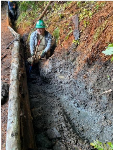
Shoveling in the muck; sawing old planks; clearing out the uphill ditch; using jacks to push up the puncheon and hold it in place – there were a lot of different jobs happening all at once.
