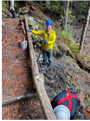
Shoveling in the muck; sawing old planks; clearing out the uphill ditch; using jacks to push up the puncheon and hold it in place – there were a lot of different jobs happening all at once.
