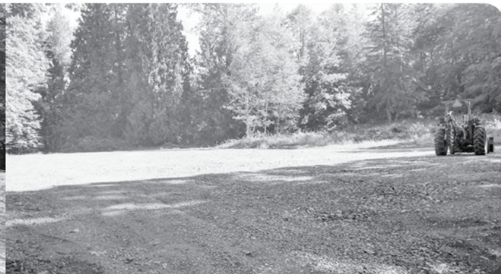
Udell parking lot, Arlington WA, 1st layer of gravel completed.
