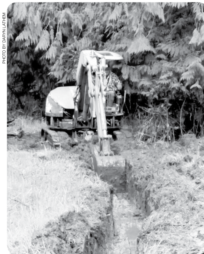
Udell parking lot, Arlington WA, drainage ditch work, Clayton Cline.
