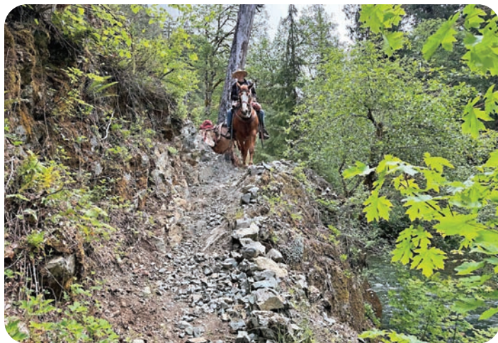
Harold Wiese testing the newly-repaired corner and drop at 5.5 miles.
