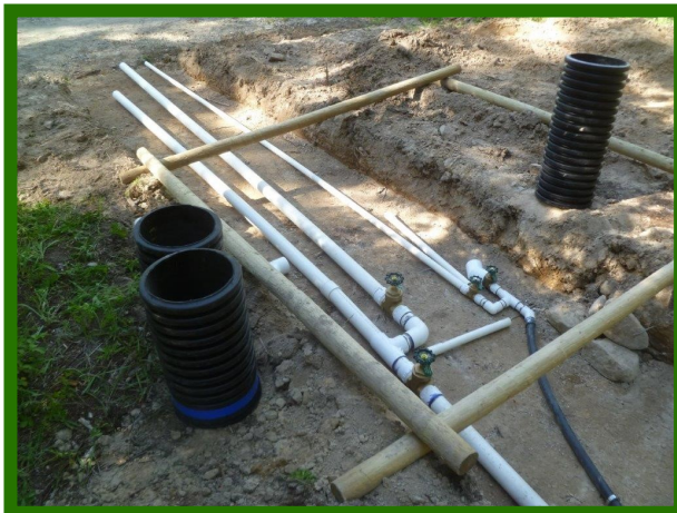
The start of the valve and drain installation at
