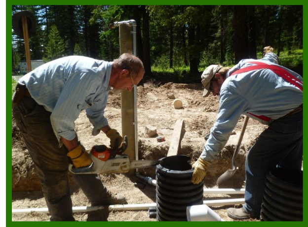
Pete (L) and Bill Ford (R) putting in covers to protect valves from fill.
