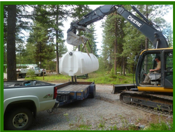
Lifting the water tank from the trailer to take it up to the hole.
