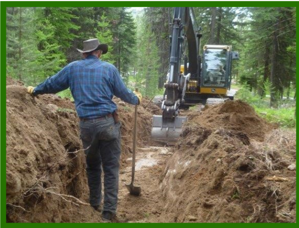
Pete and Jeff digging trench for pipes between tank and the inlet and outlet.
