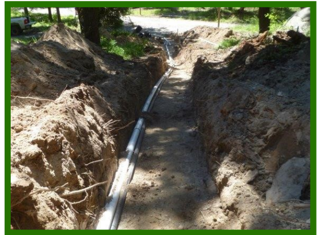
280 ft of 3 inch PVC and one and half inch black plastic laid in trench. (View is from tank end.)
