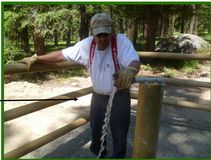
The water outlet compound that allows proper drainage is ready for the gate.
