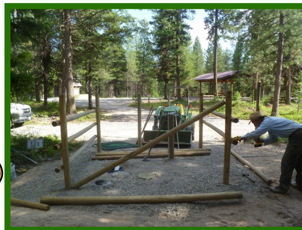
Pete installing fence around water outlet.
