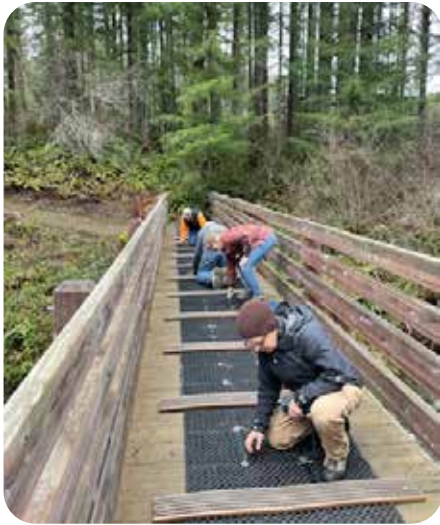
Setting mats on bridge.
