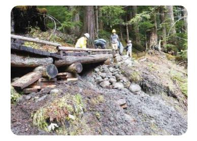
Shoveling in the muck, sawing old planks, clearing out the uphill ditch, using jacks to push up the puncheon and hold it in place – there were a lot of different jobs happening all at once. Rocks had to be collected. Off-site drainage work needed to be done.
