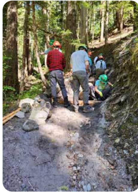
WTA crew installing check step on Toutle Trail
