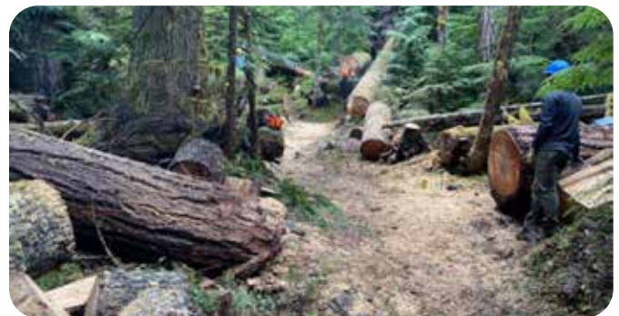
Finishing touches – angling the logs to the lay of the trail.
