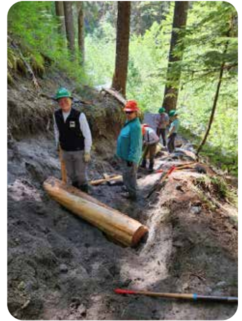
WTA crew installing check step on Toutle Trail
