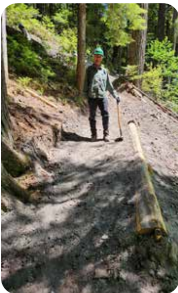
WTA crew finished curb rail on Toutle Trail
